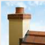
Brick or Stone Chimney (Class 1)
